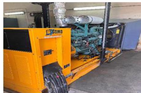
Fig. 4 Real view of the power generator 500KVa
