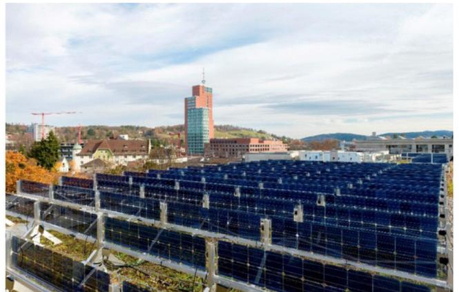
Fig. 3. Example of a vertically mounted BPV system on a green roof in Winterthur, Switzerland [7].
