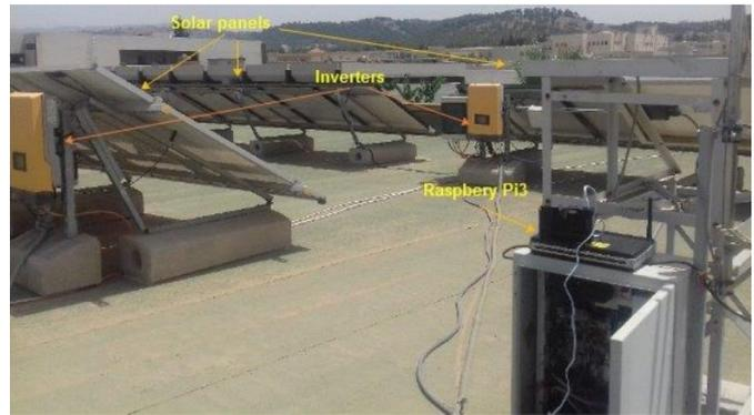
Fig. 5. A wireless prototype for monitoring solar PV systems [5].
